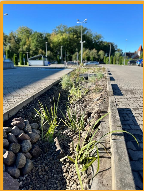
Rain garden in the parking lot
