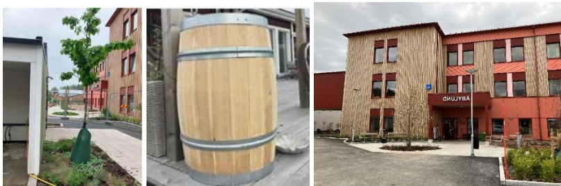
Housing company Reuse of rainwater for flushing toilets Gamleby
