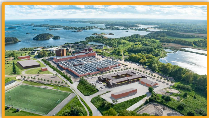
The Water Recycling Plant Kalmarsundsverket in Kalmar / Sweden
