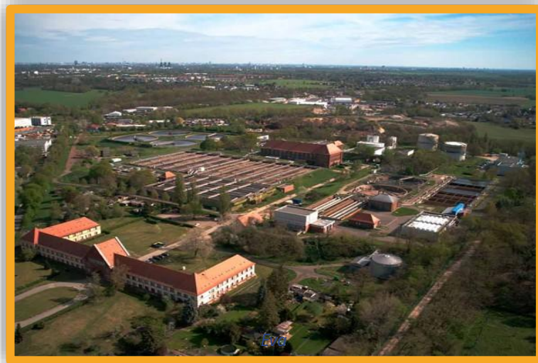
WWTP Stahnsdorf south of Berlin / Germany
