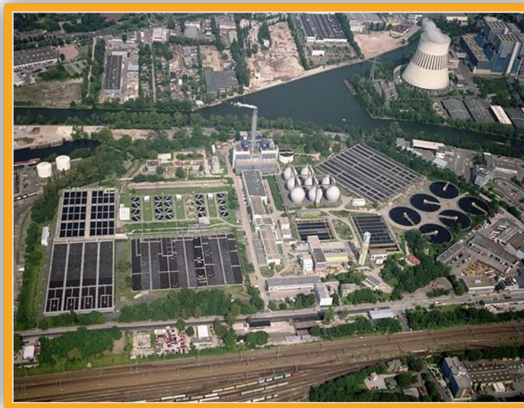
WWTP Ruhleben in Berlin / Germany
